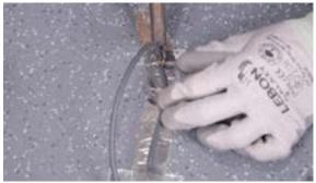
**Step 5)** Remove the protective tape from the sides and using the Mozart Weld Trimmer with the 0.7mm spacer in place, trim the weld and allow to fully cool. If the working area is warm, use a cloth with cold water to cool the weld quicker.
