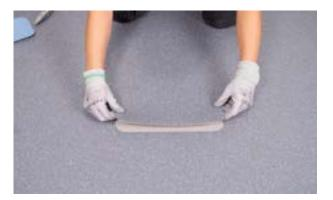
**Step 5)** Ensuring the correct orientation, place the new piece into position. Carefully trim to fit.
