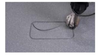
**Step 10)** When approaching the end of the repair, take care to run the weld into the "V" cut and control it so it says on line. At the end of the "V" cut, continue over the 5mm of exposed weld and pull away the weld gun.
