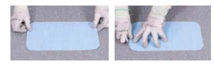
**Step 2)** Place the template over the damaged area. Using a straight knife, carefully score around the template edge.
