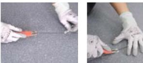
**Step 7)** Remove the protective tape and trim the weld cord flush using the Mozart Weld Trimmer with spacer retracted.
