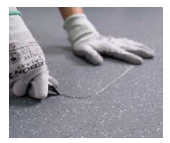
**Step 3)** Remove the template and use the hooked knife to cut through the score line enabling the damaged area to be removed. Remove and debris from the subfloor.
