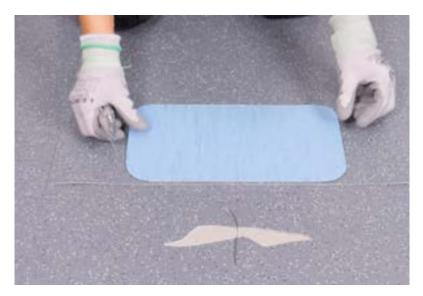
**Step 1)** Create a template from old flooring or another solid material. This can be re-used and keeps all repairs a consistent size. Always round off the corners, this ensures the weld can be completed in one.
