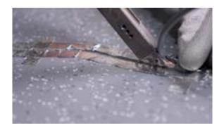
**Step 4)** Apply the weld cord through the nozzle and into the damaged area. Ensure constant movement, pressure and speed.
