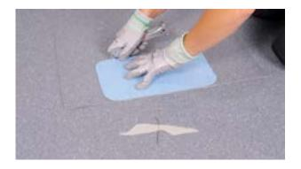
**Step 4)** Place the template onto a new piece of flooring and repeat the process of scoring and cutting.
