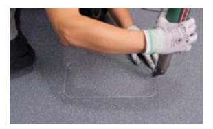
**Step 8)** Using a welding gun with the Turbo Roller Nozzle attached, set the temperature to 7 and allow to warm. Apply the weld cord through the nozzle and start to run along the groove. Ensure constant movement, pressure and speed.
