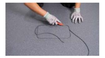
**Step 11)** Using the Mozart Weld Trimmer with the spacer retracted, trim flush the weld to the surface of the flooring.
