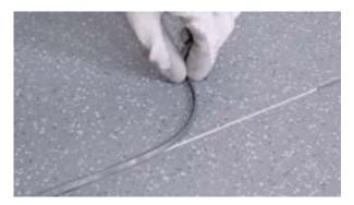
**Step 1)** Remove all the loose weld cord up to where the remaining cord is well fused. Carefully cut so the old material can be disposed of. Check the exposed groove to ensure it is free from debris.
