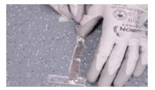
**Step 2)** Use the aluminium or masking tape to contour the perimeter of the damaged area.
